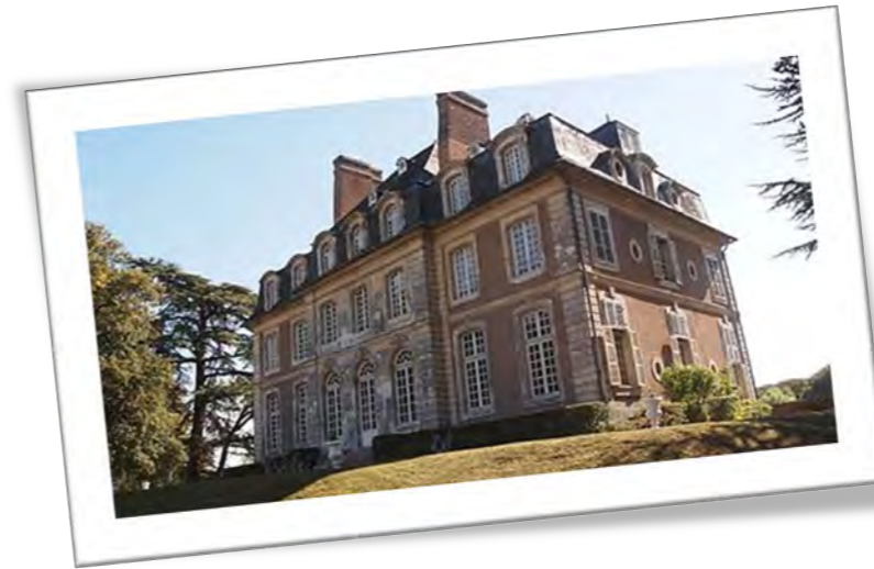
PHOTO 19 - CHATEAU DE REVERSEAUX – FAÇADE NORD (WIKIPEDIA)
